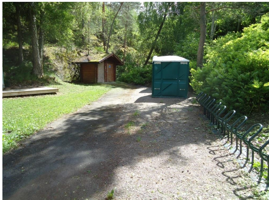
Figur 42 Handicaptaolettet skal rives. Kilde: COWI AS 2017
